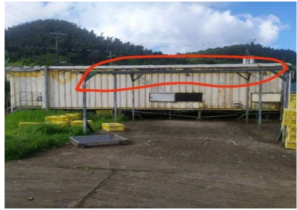
Figure 5. poultry holding pen to be renovated
