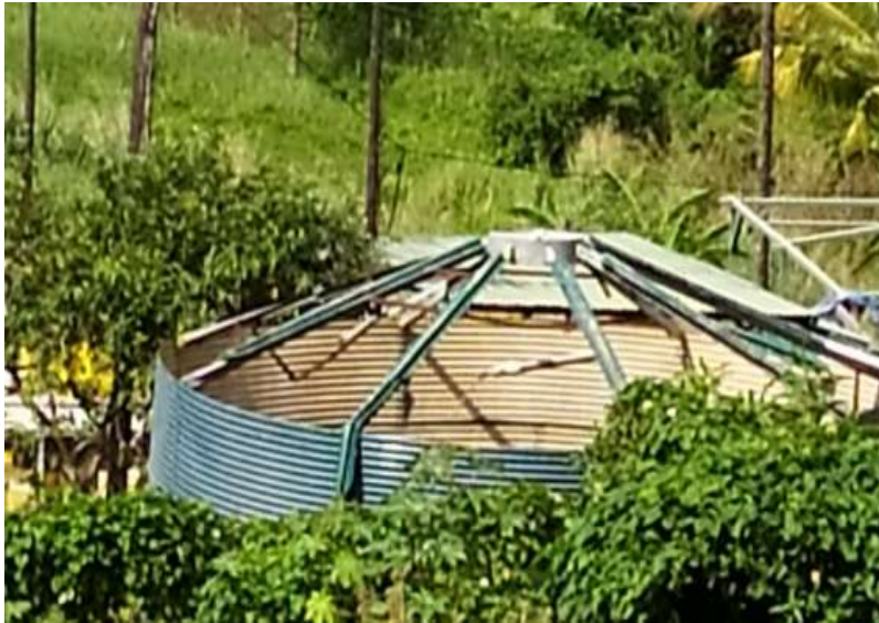
Figure 12: Water storage tank
