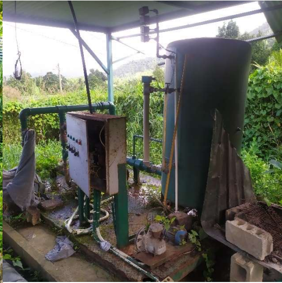
Figure 18. Chlorination tank
