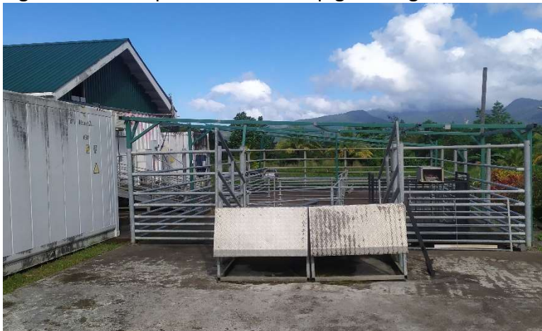
Figure 9. Roof replacement of the pig holding shed
