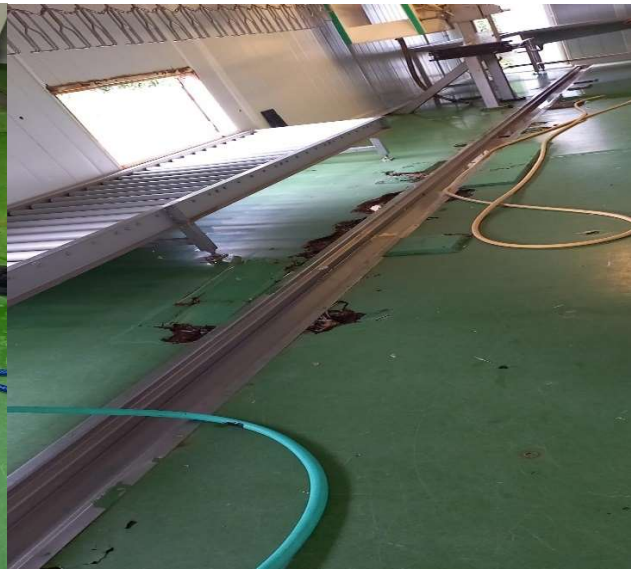
Figure 6 and 7. Damage wooden floors to be replaced with zinc metal sheet
