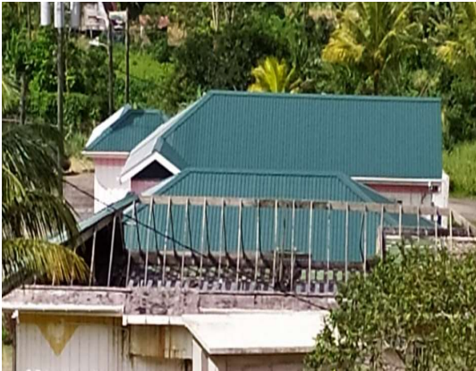
Figure 4: roof of poultry slaughterhouse
