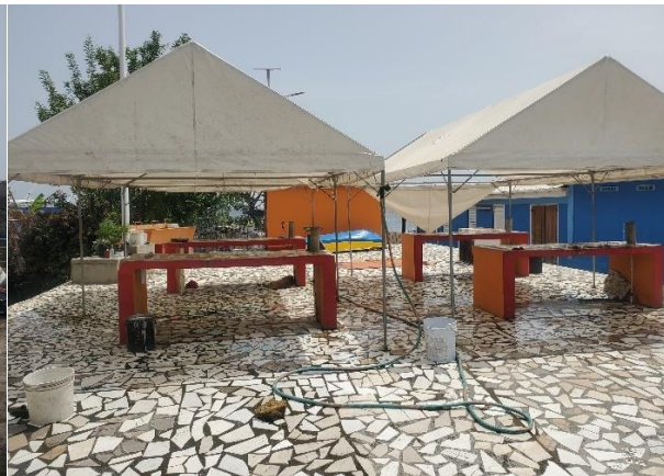
Photo 2. Concrete roof to replace tent
