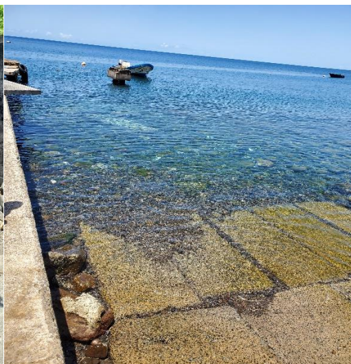
Figure 2. Slipway to be rehabilitated
