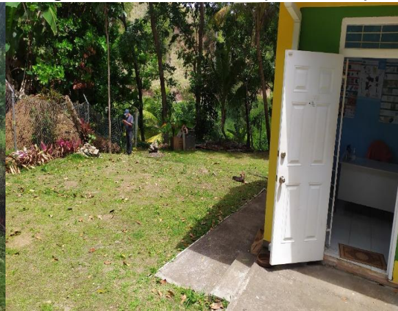
Figure 2. Extension area (front view)
