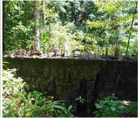
Photo # 2. Bridge to be repaired
