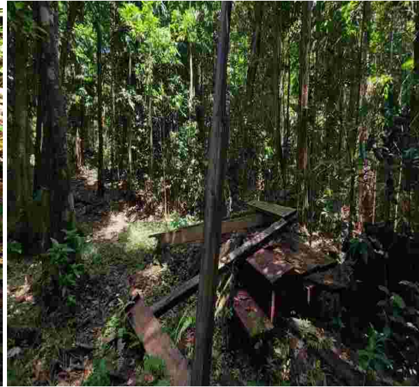
photo # 6. Gazebo to be replaced
