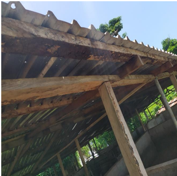
Photo # 1: Roof repairs to be done
