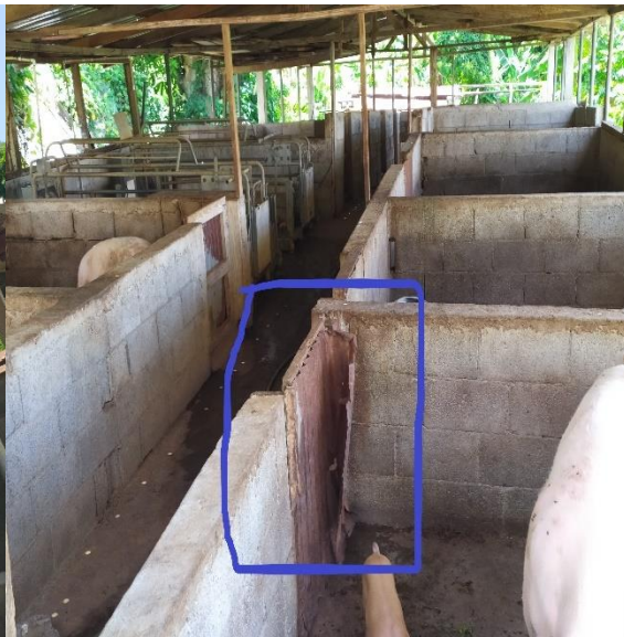
Photo # 2: Replace doors
