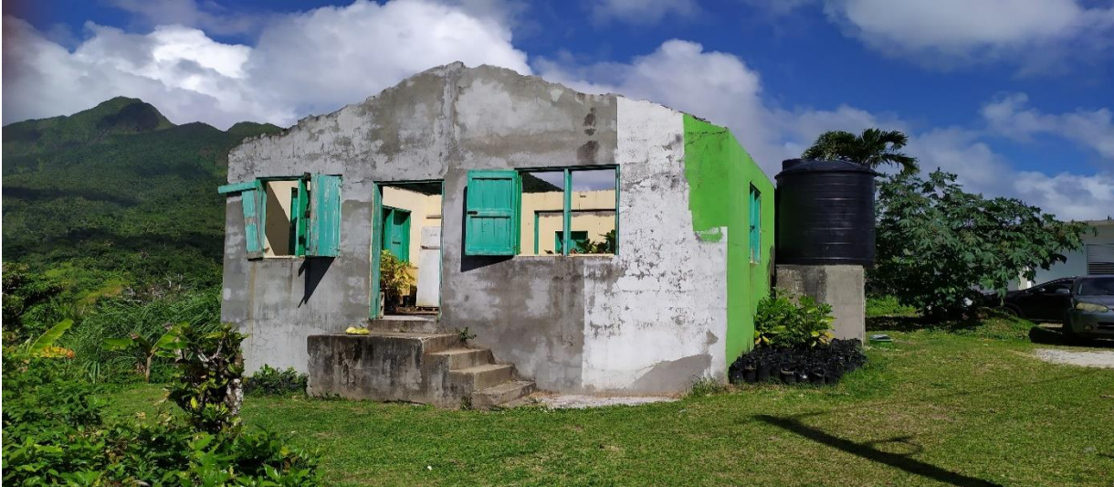
Figure 2: Baseline condition of Delices Forest Service Centre (exterior)
