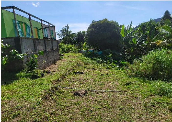
Figure # 4. Area to be backfilled.
