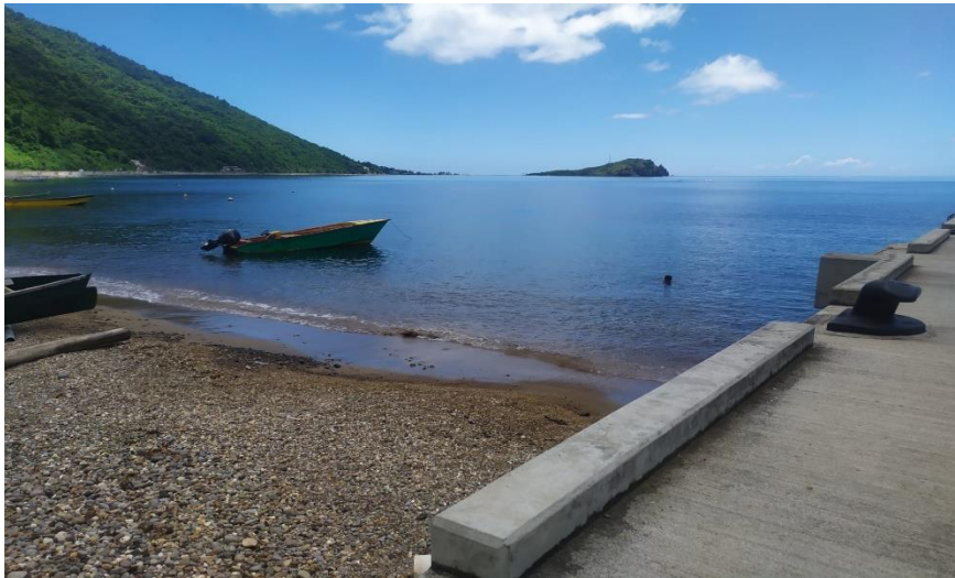
Photo 2. Proposed site for slipway at Soufriere Landing Site
