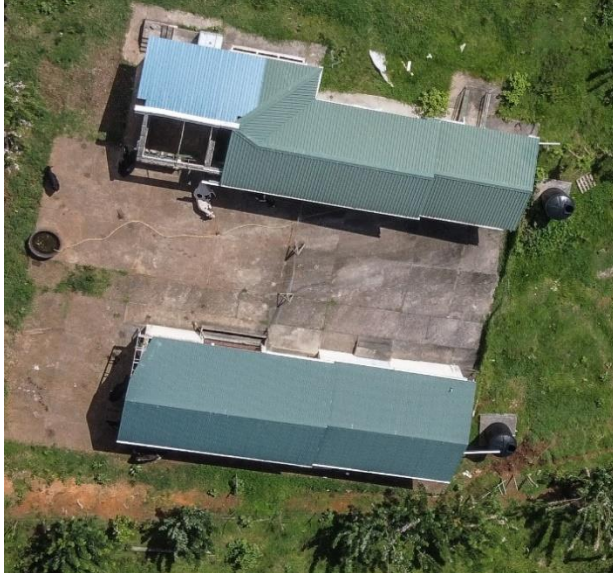
Figure 4: Existing Dairy Parlour
