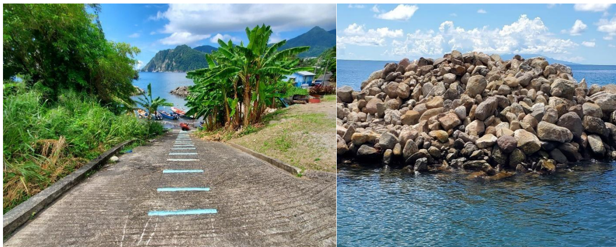
Photo # 7. Slipway gliders to be replaced
