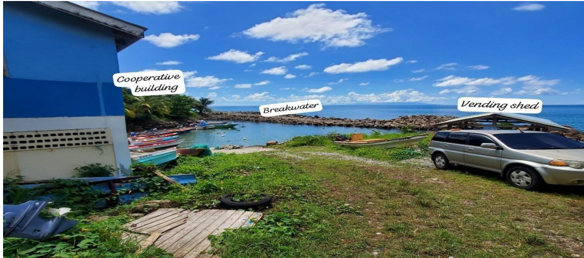
Photo # 4. Location of cooperative and vending building in relation to breakwater
