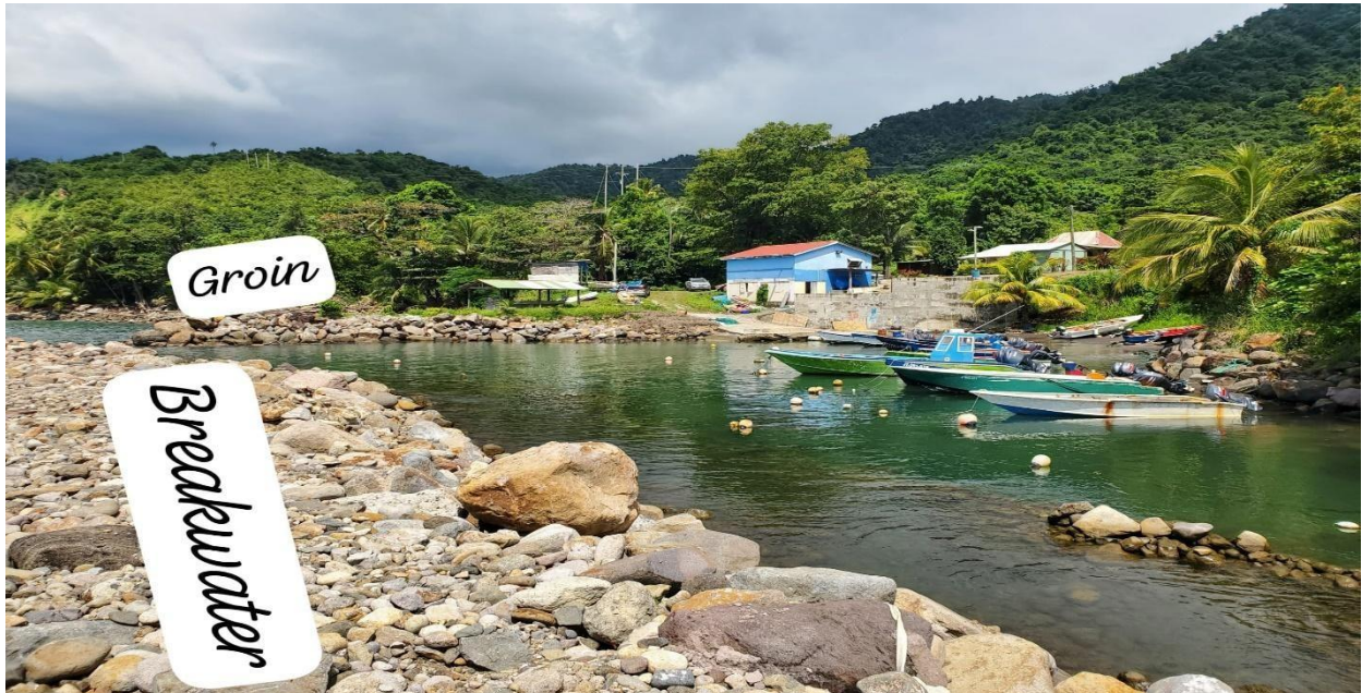
Photo 1. Breakwater (parallel to shoreline) and Groin (perpendicular to shoreline) at Stowe
